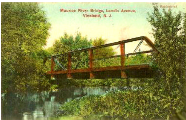
Maurice River Bridge, Landis Avenue, Vineland, NJ
